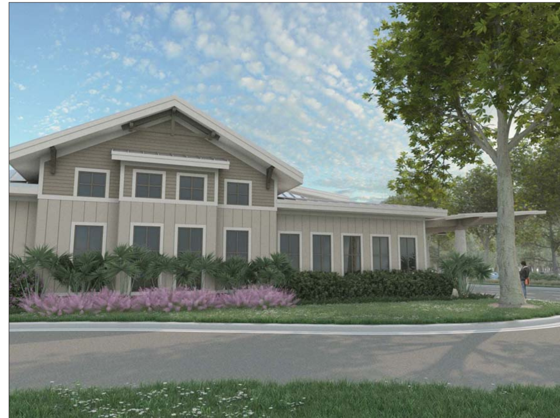
VIEW AT BAG CLAIM END OF TERMINAL
