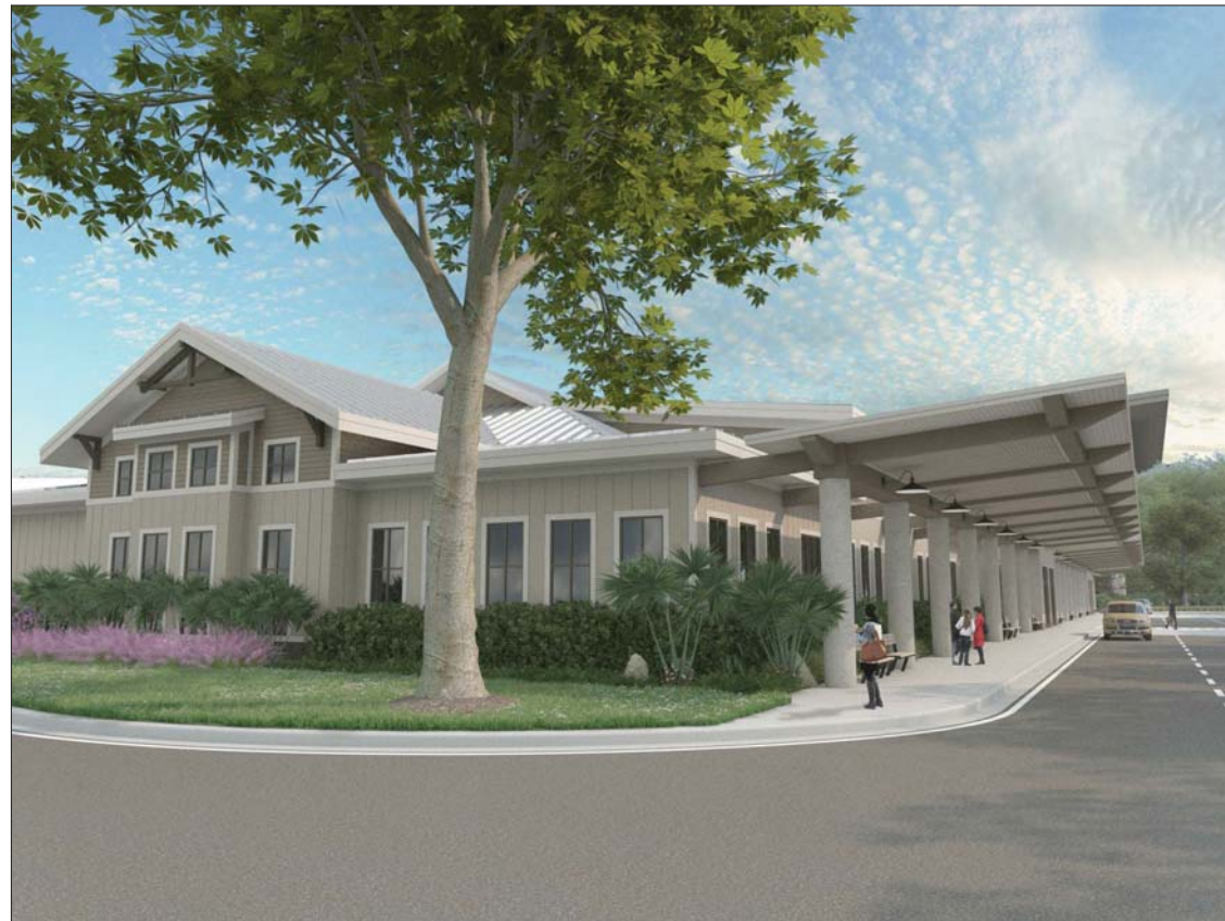
VIEW AT BAG CLAIM END OF TERMINAL
