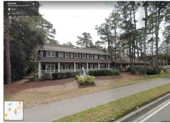
FACADES ACROSS W.M. HILTON PARKWAY FROM SUBJECT PROPERTY
