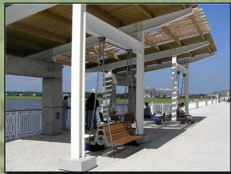
PIER SHADE STRUCTURE
