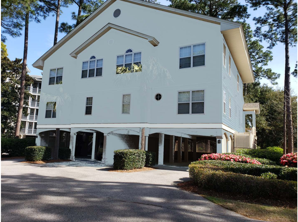
Figure 1. Lyons building from Wimbledon Ct
