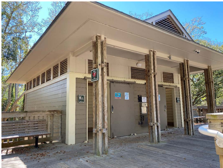
Image of the existing toilet facility at Islanders Beach Park. Colors and materials will match this toilet facility.
