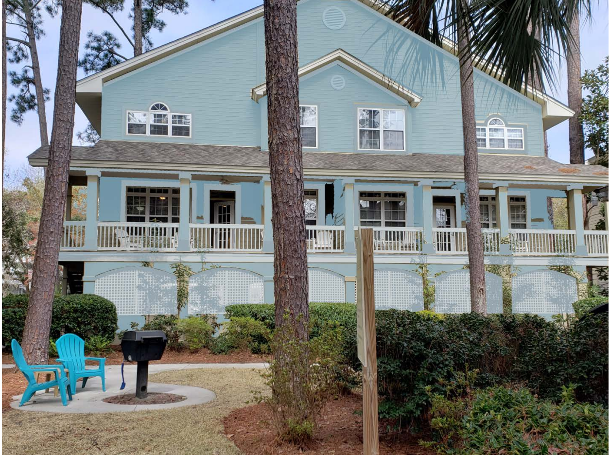
Figure 3. Lyons building front (from pool view)
