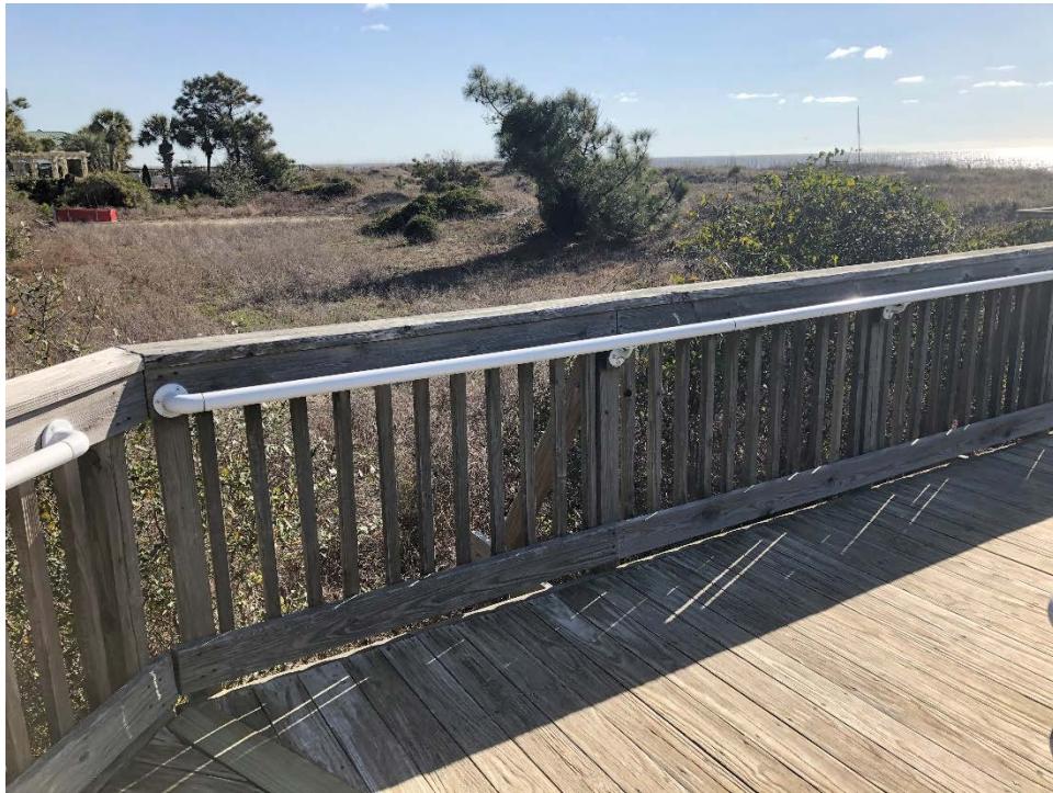
Location of future Overlook off existing boardwalk. Guardrails at New Overlook will be similar in style and construction as existing boardwalk guardrails.
