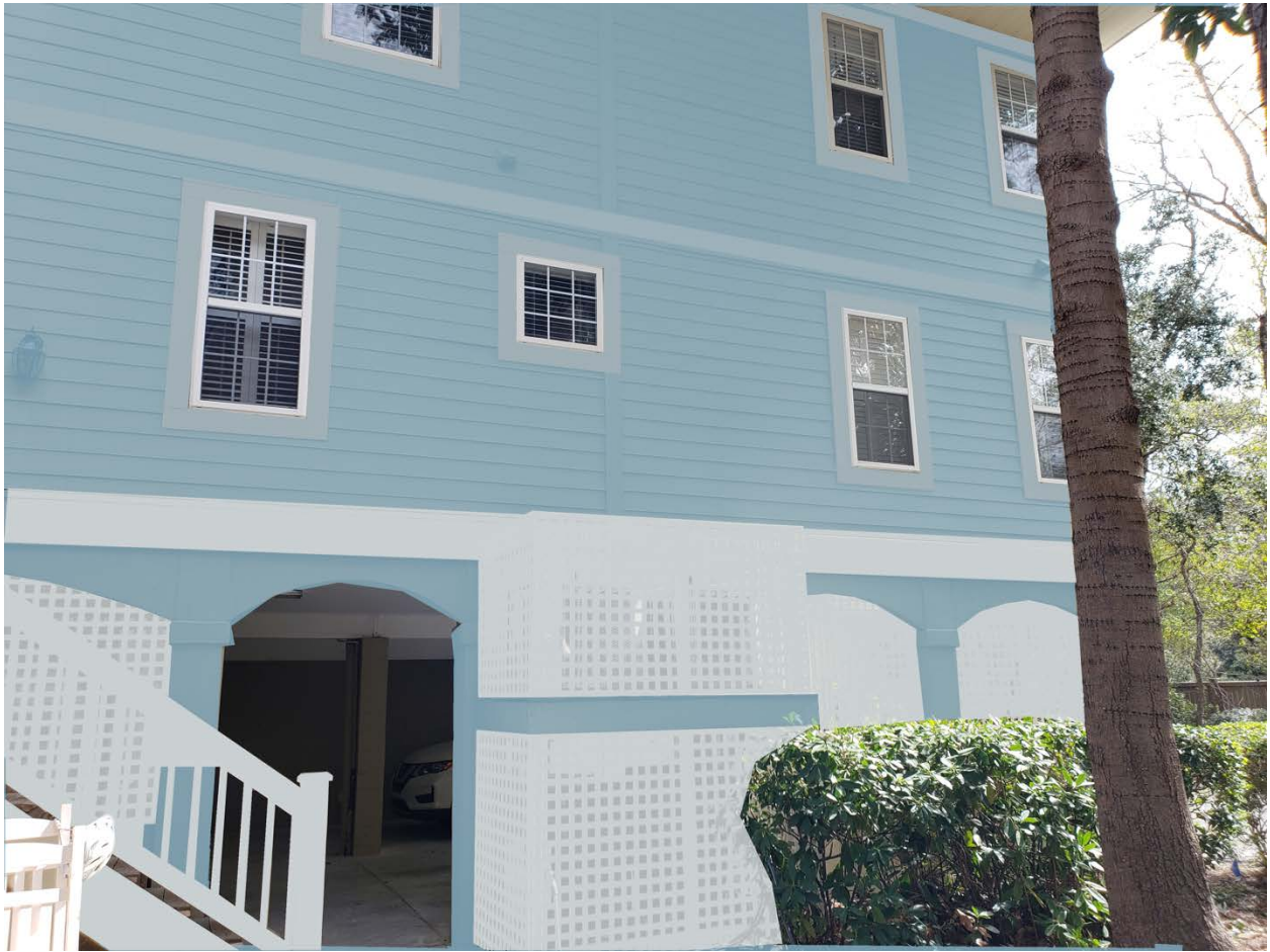
Figure 2. Lyons building - side view
