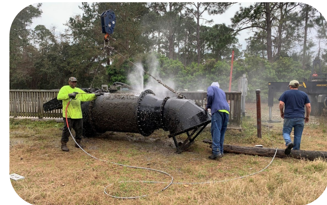
Pump Maintenance (Wexford Station)
