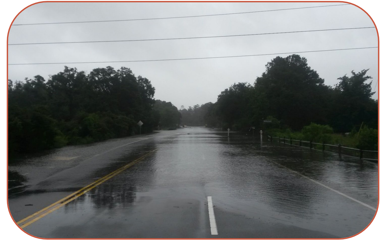
Hurricane Irma storm surge at Mathews Drive
