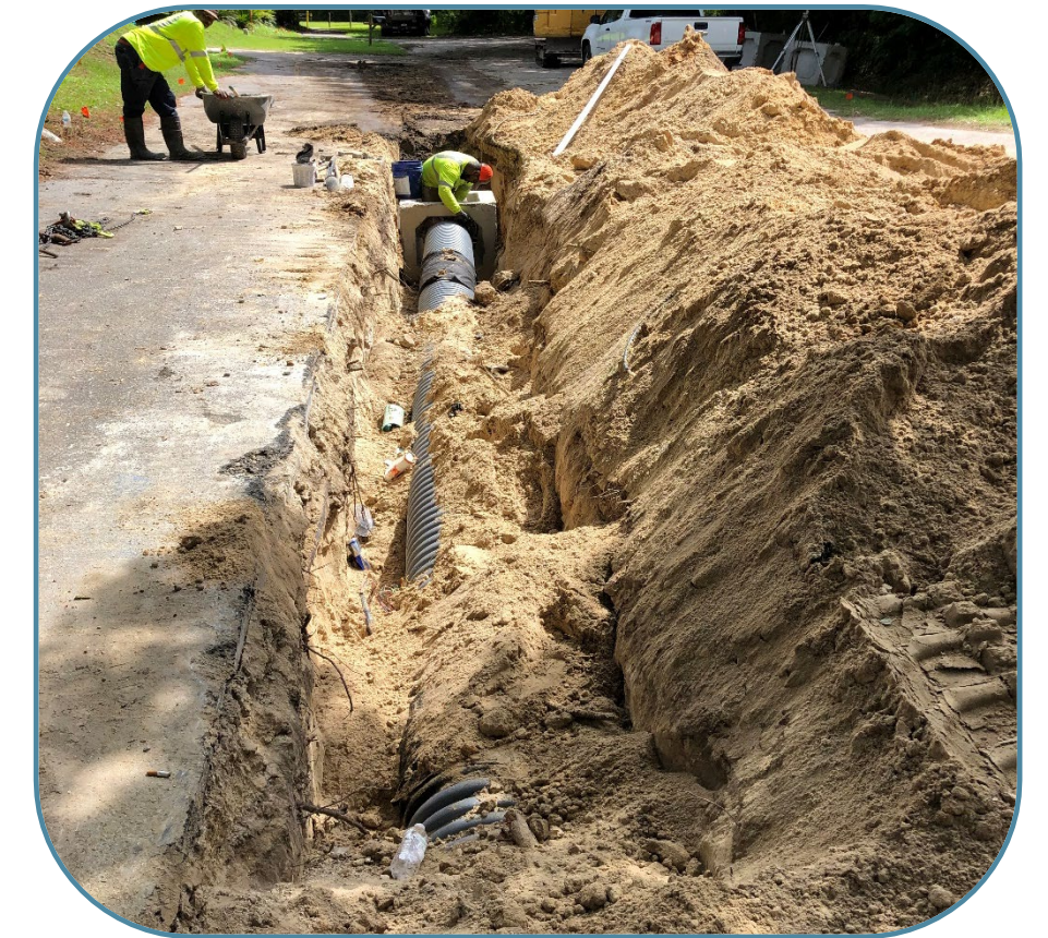
Pipe Installation (Old Wild Horse Road)
