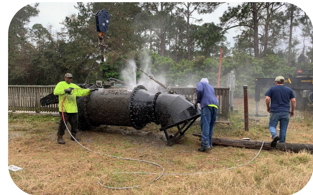
Pump Maintenance (Wexford Station)
