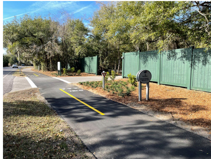
Pathway Relocation – Beach City Road
