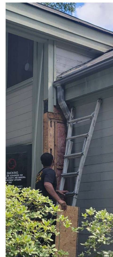
Figure B-1: Building D siding repair, March, 2022
