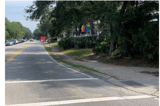
Wood Bridge Repair – Gardner Drive
