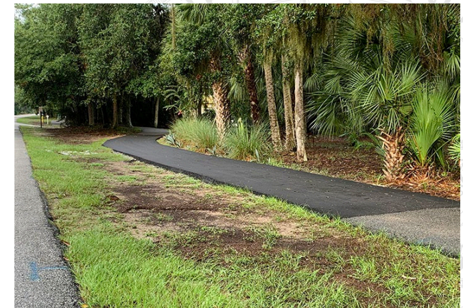
Asphalt Replacement - North Forest Beach
