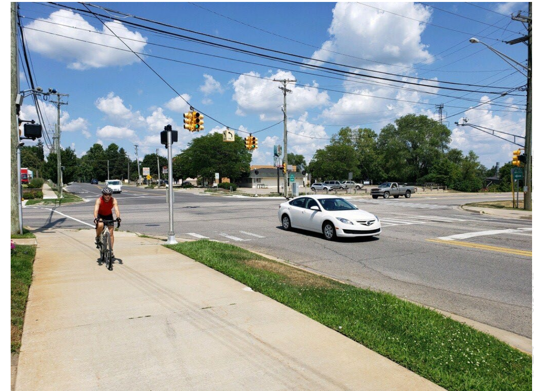
Adaptive Traffic Signals
