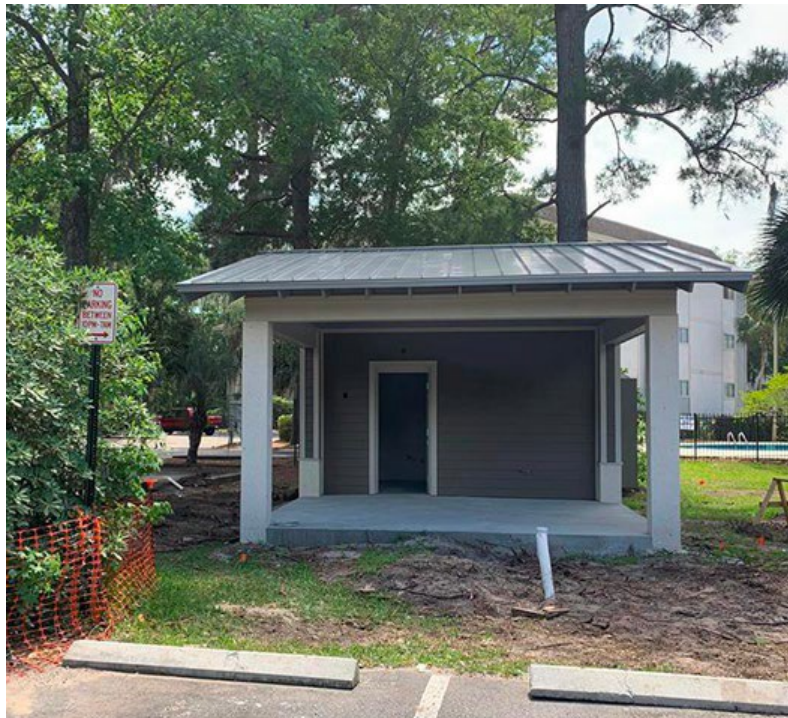
Cordillo Tennis Courts Restroom Building
