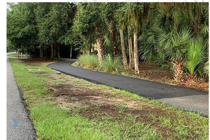
Asphalt Replacement - North Forest Beach
