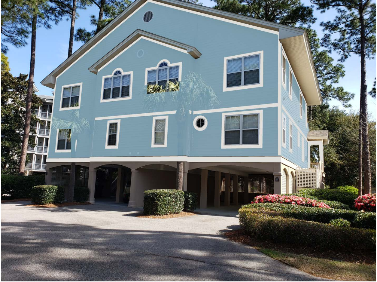
Figure 3. Rear of Lyons building (facing road) showing proposed color and trim.
