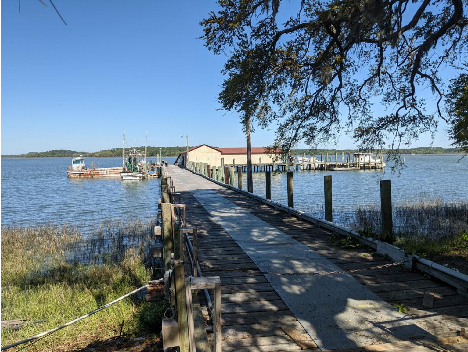
EXISTING DOCK (PROCESSING BUILDING TO BE DEMOLISHED)
