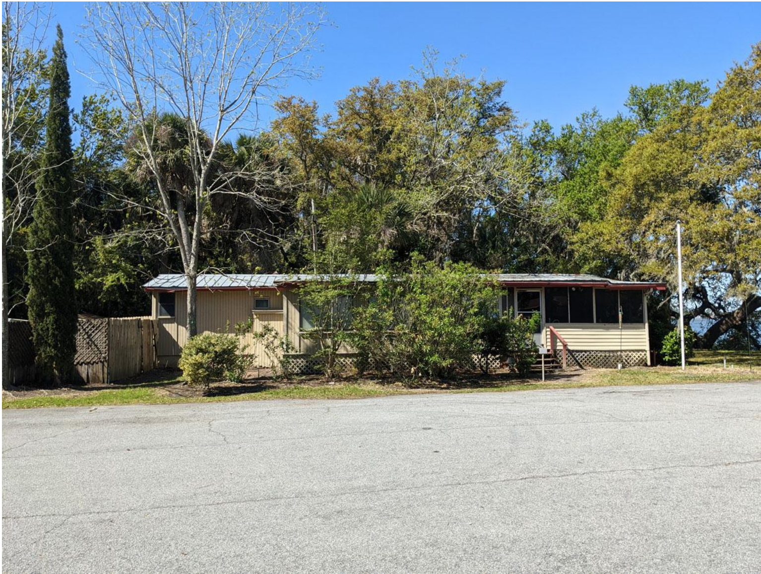
EXISTING MANUFACTURED HOME (TO BE DEMOLISHED)
