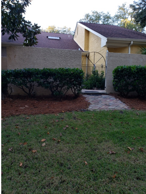
Figure 8. Beckingham (Neighboring Building)
