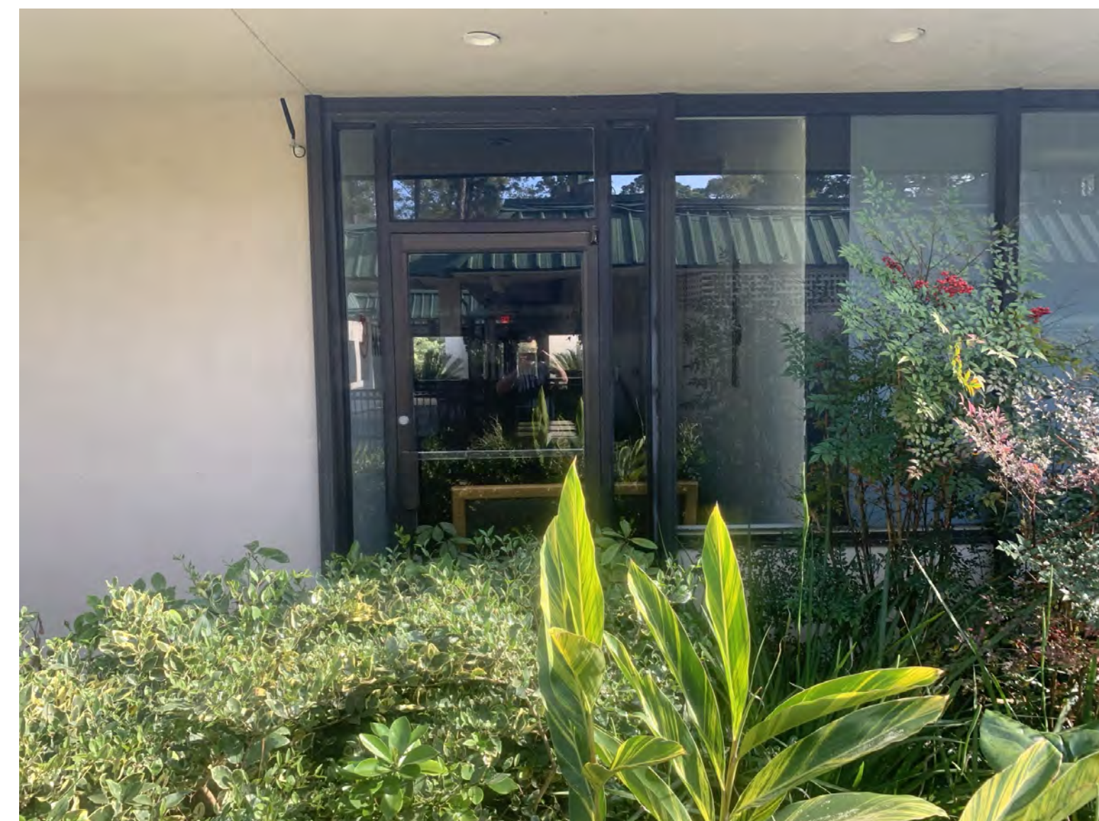
DOOR TO BE REMOVED
