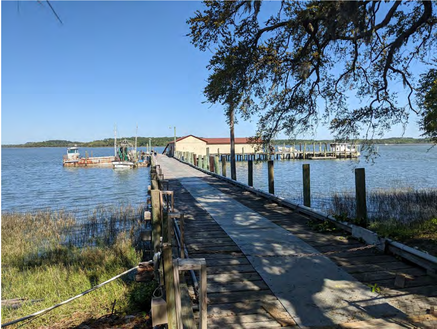
EXISTING DOCK (PROCESSING BUILDING TO BE DEMOLISHED)
