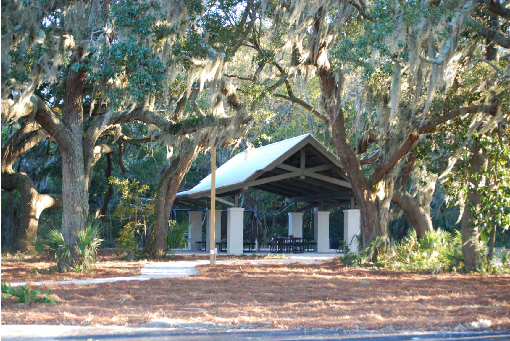
ROWING & SAILING CENTER (GALVANIZED ROOF APPROVED IN 2013)
