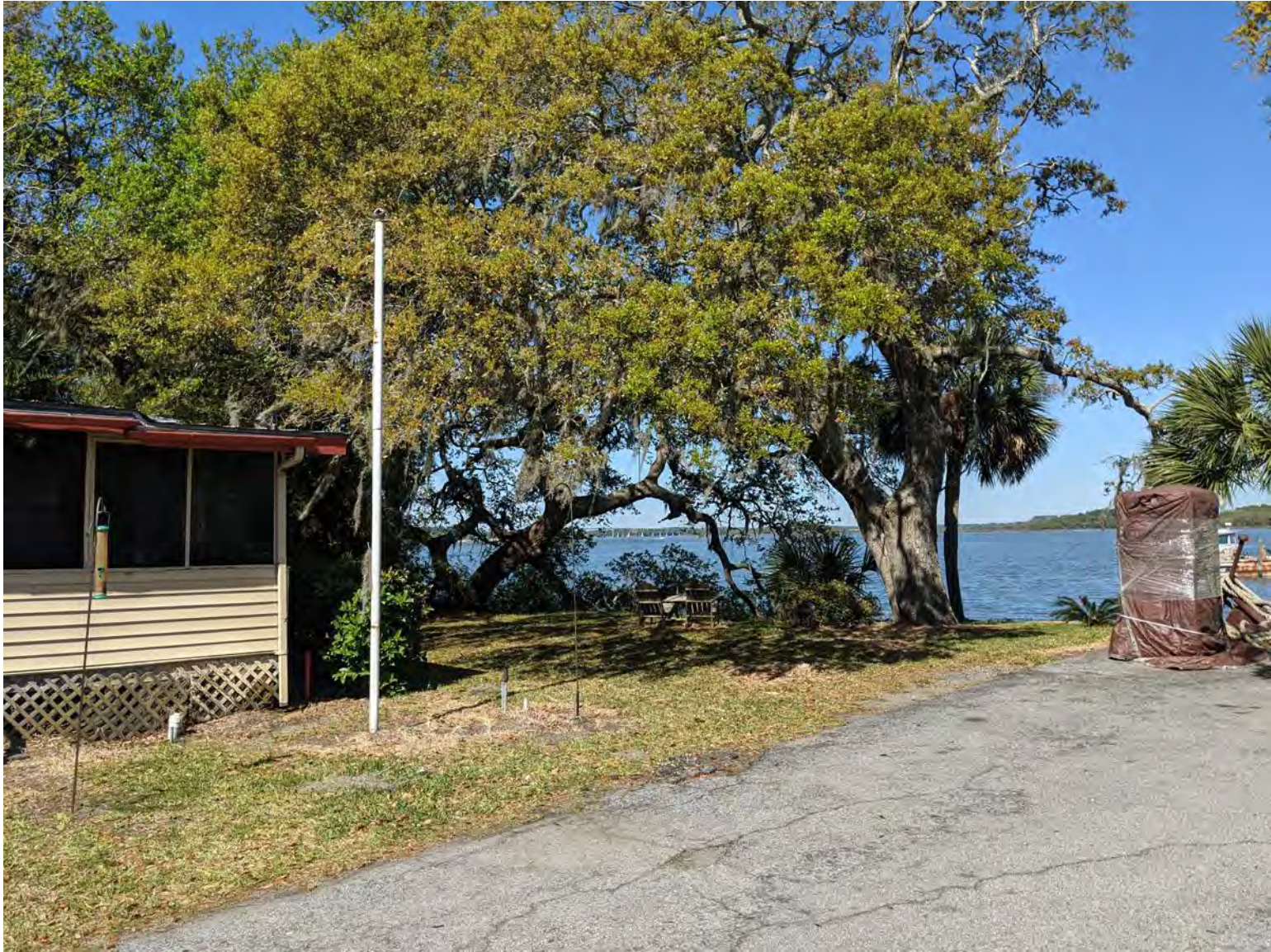
EXISTING MANUFACTURED HOME (TO BE DEMOLISHED)
