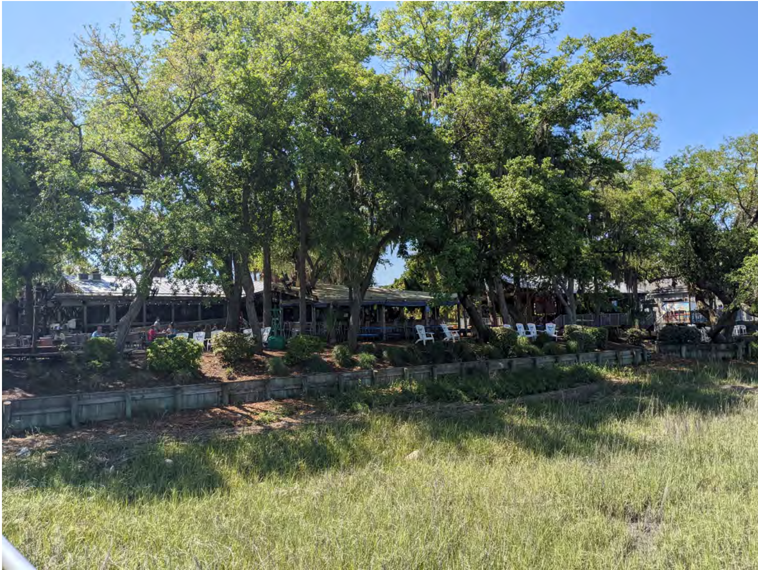
SKB RESTAURANT & DOCKSIDE'S BAR (GALVANIZED ROOFS)
