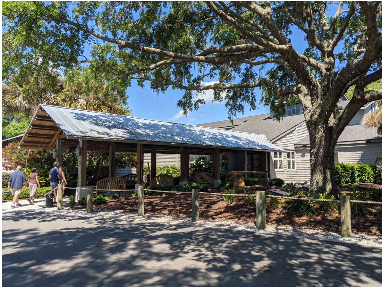
DOCKSIDE RESTAURANT (GALVANIZED ROOF APPROVED IN 2017)
