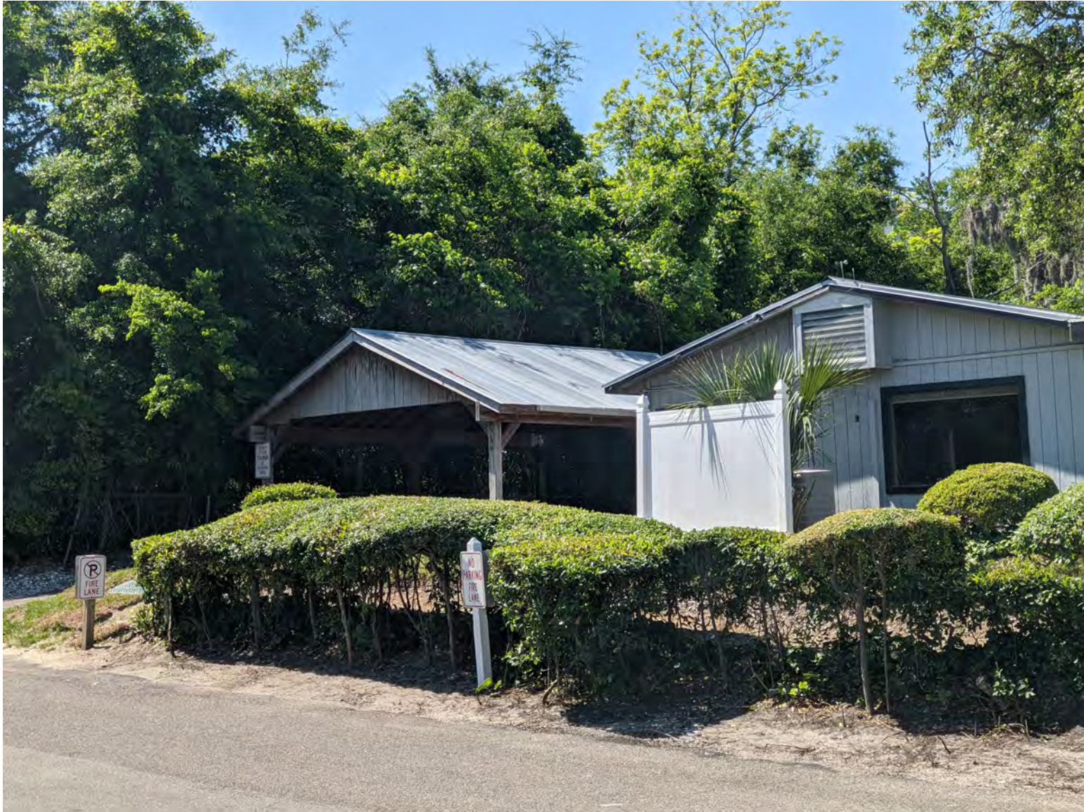
I HUDSON RD. - CARPORT ADJ. TO HUDSON'S (GALVANIZED ROOF)
