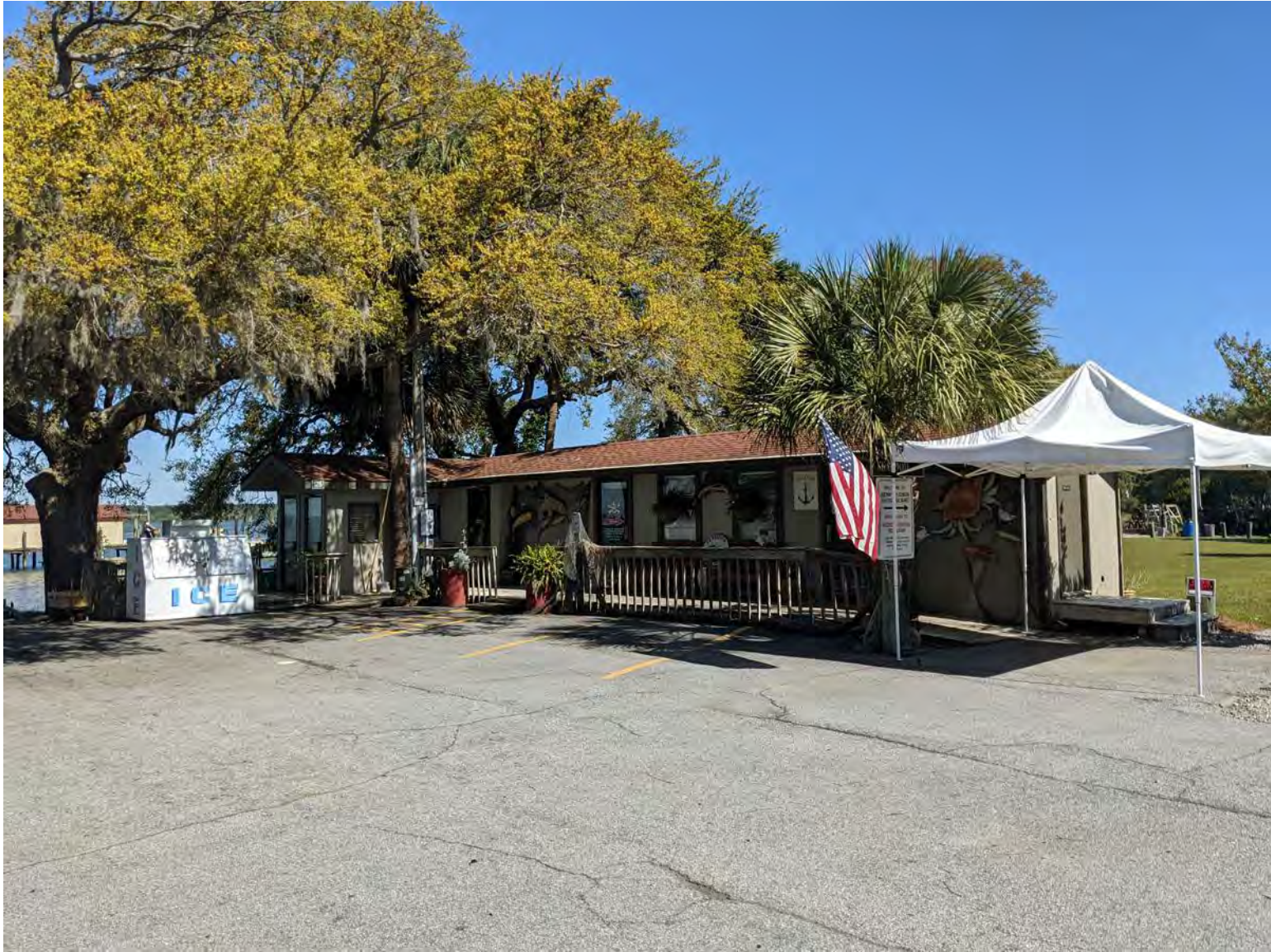
EXISTING BENNY HUDSON SEAFOOD MARKET (TO BE DEMOLISHED)
