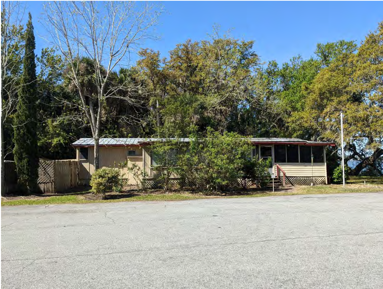
EXISTING MANUFACTURED HOME (TO BE DEMOLISHED)
