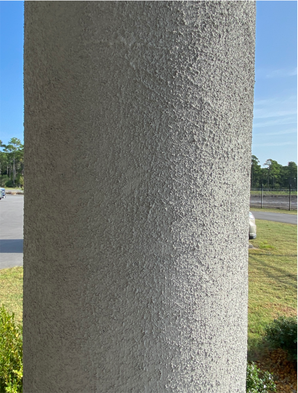
Actual installation of the proposed acrylic coating on a concrete column.
