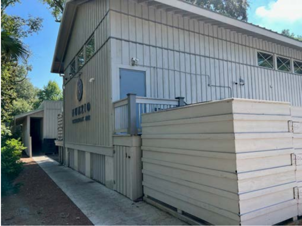
Rear of building at new service yard location
