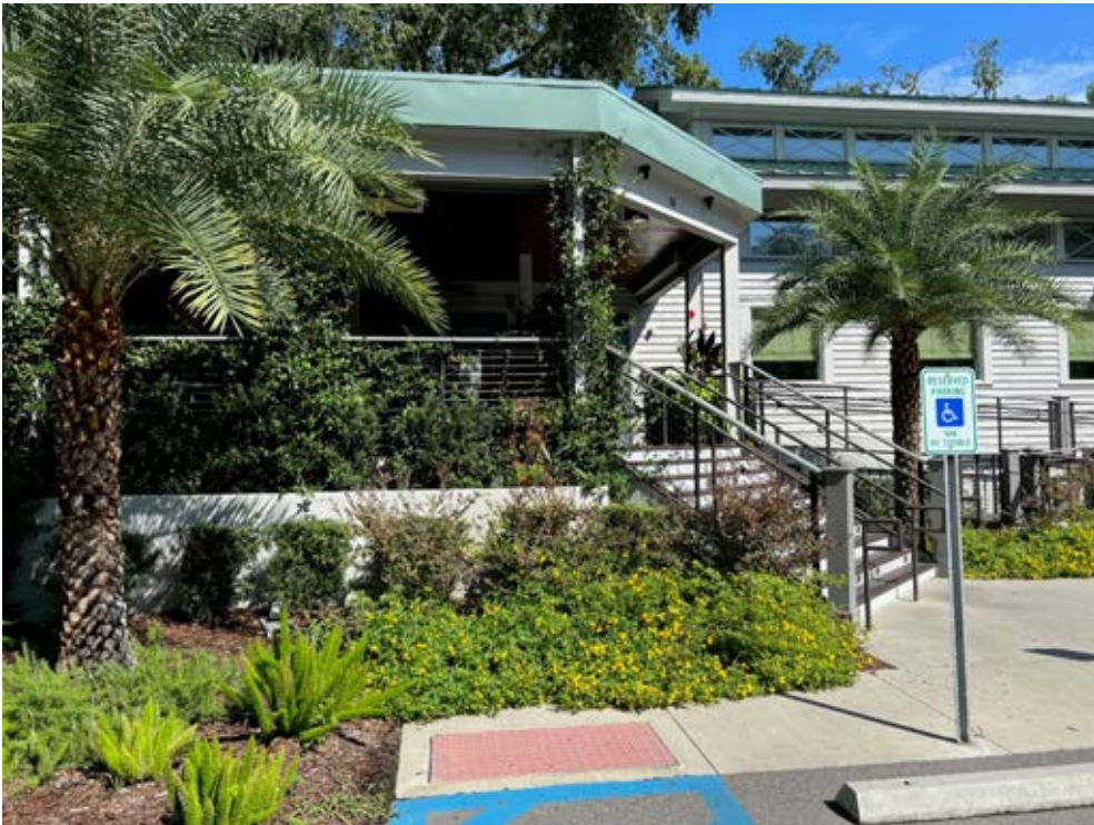
Front of building with jasmine
