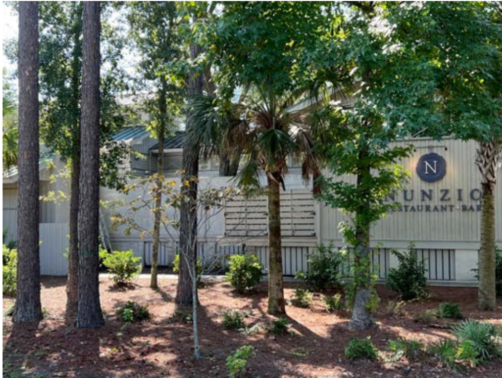
Existing facade facing highway 278
