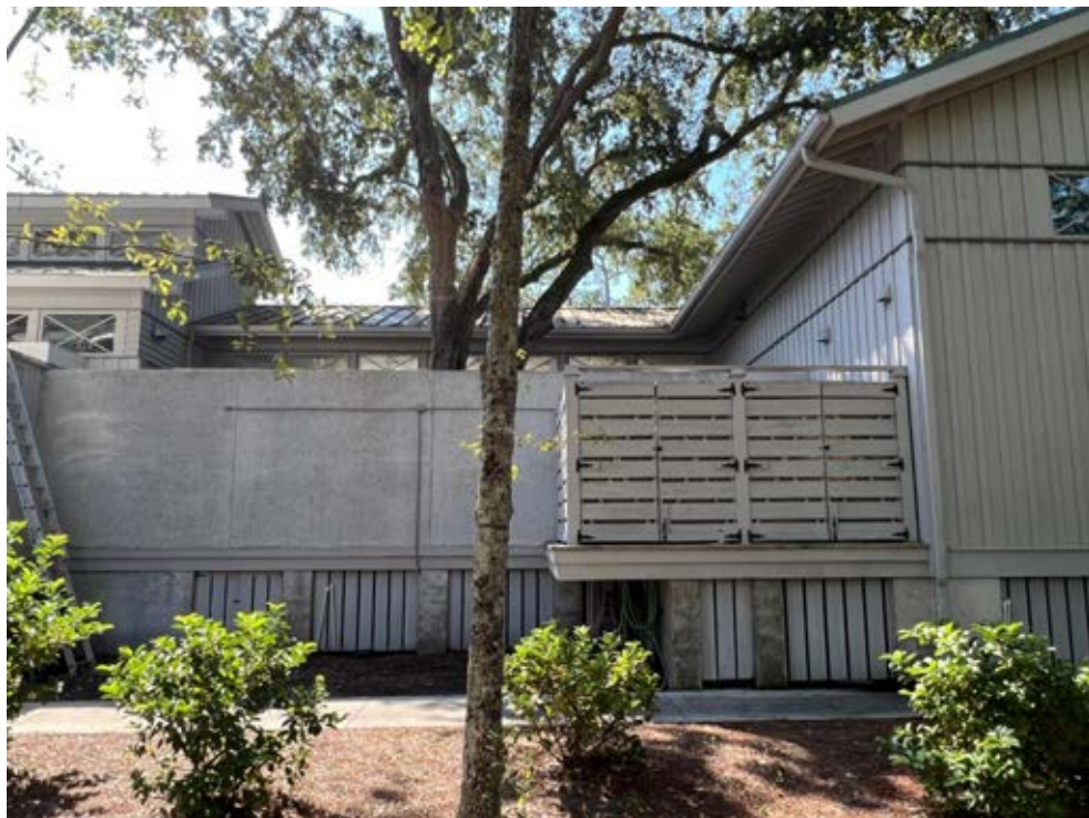
Rear deck area enclosed by wall
