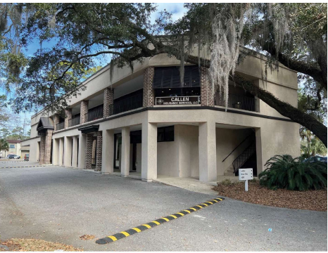
EXISTING PARKING LOT SIDE PHOTOS
