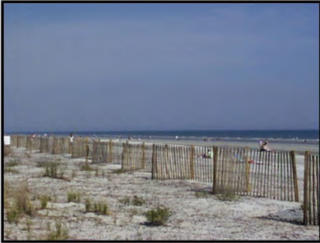
Figure 27: Sand Fencing on Hilton Head Island.
