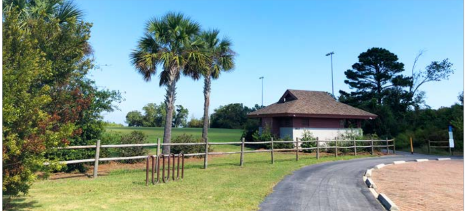
Barker Field Extension restroom building and parking with pathway
