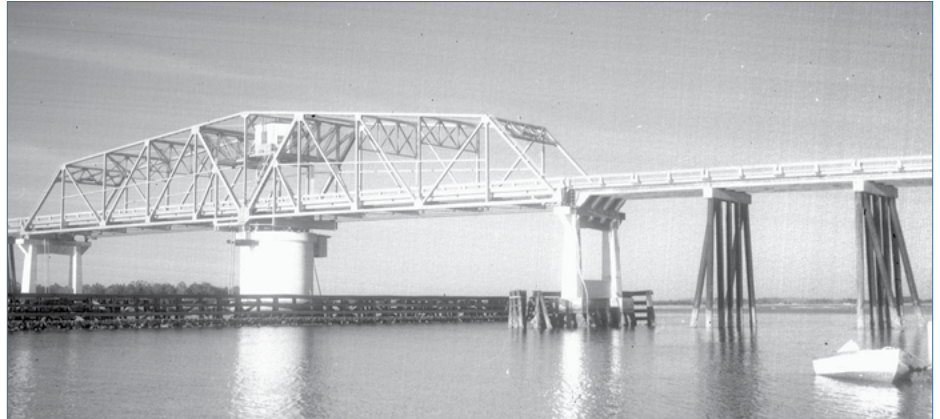
The two-lane swing bridge to the Island was replaced in 1982.
