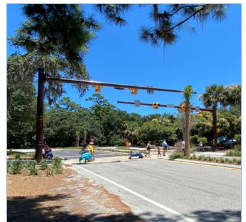
HAWK signal at Coligny Circle
