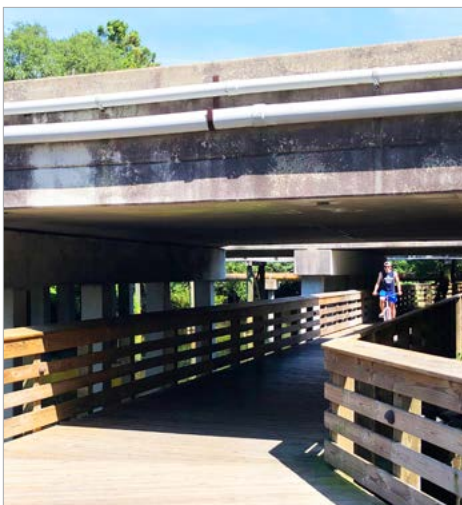
The underpass on U.S. 278 provides safe crossing for pathway users.
