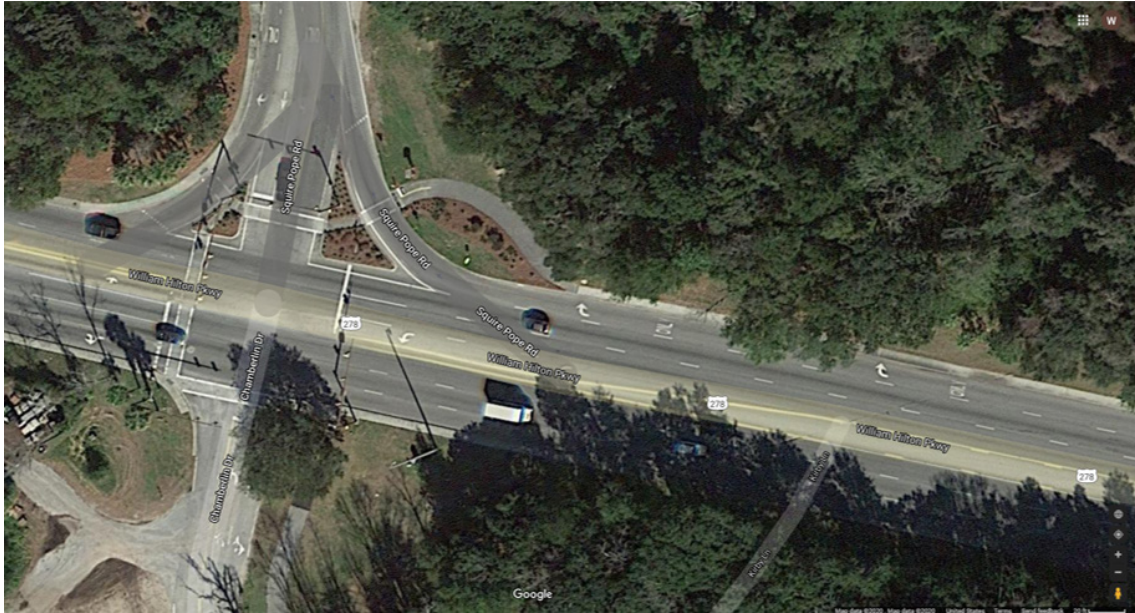
Image 4.6: Pathway along William Hilton Parkway without horizontal separation from the roadway.
