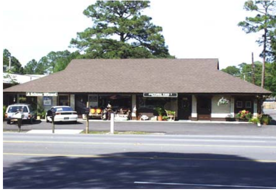
Existing Non-Conforming Structure - Palmetto Bay Road
