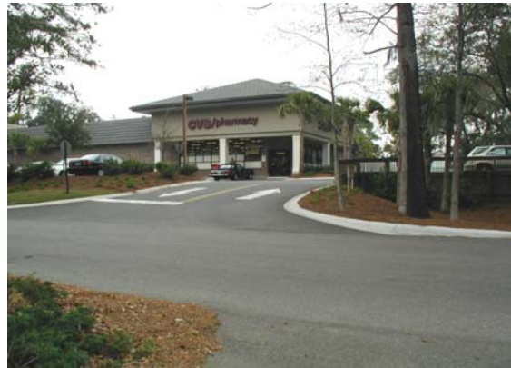
Dry floodproofed Structure (substantial soil fill).
