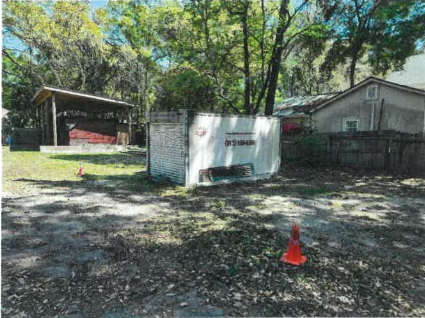
Existing Structure – Shed
