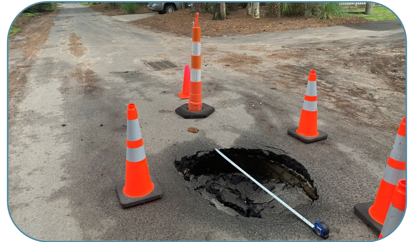
Pipe joint failure causing sinkhole in roadway
